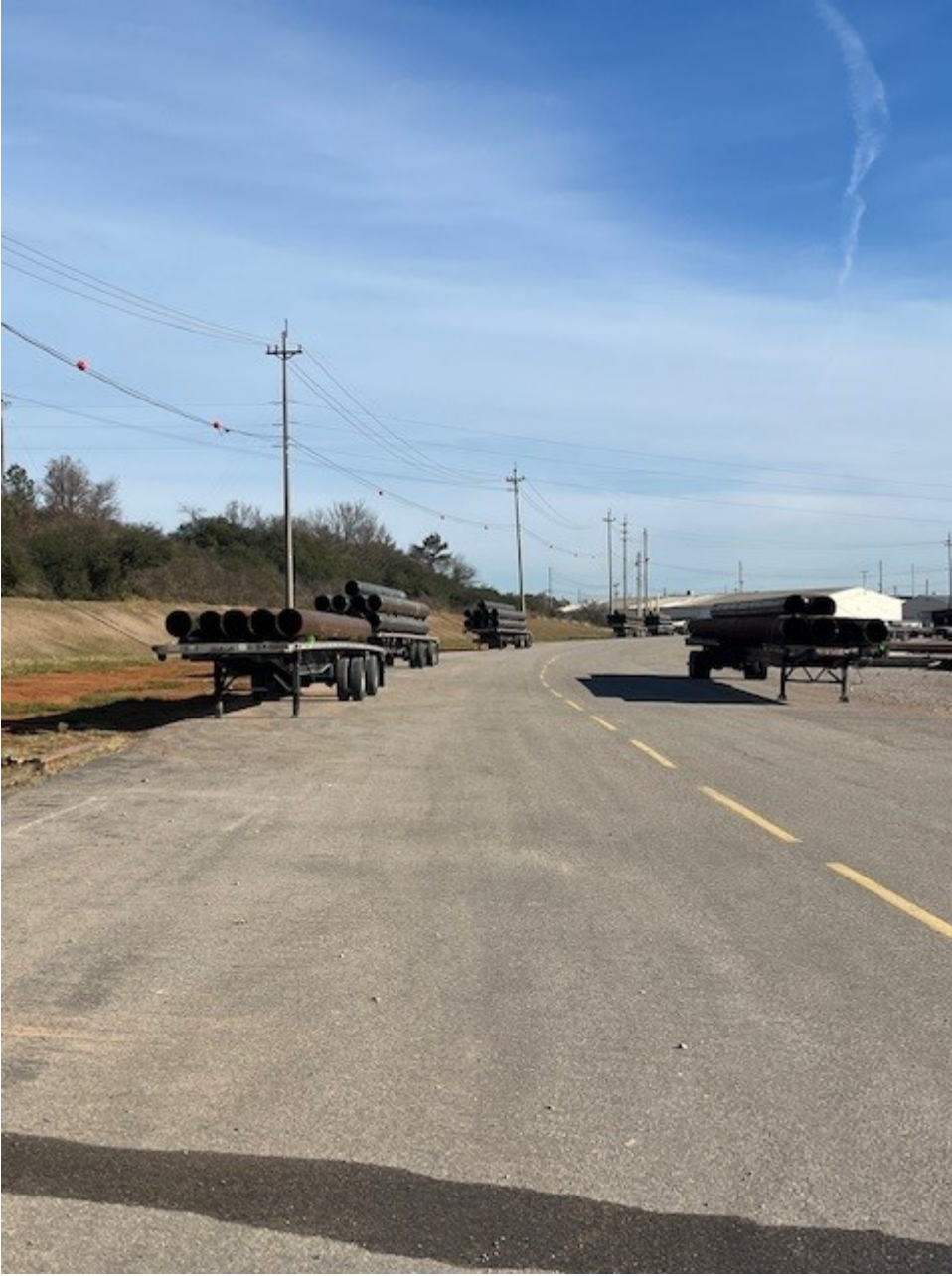
Preloaded trailer are normally lined up on each side of the road.
